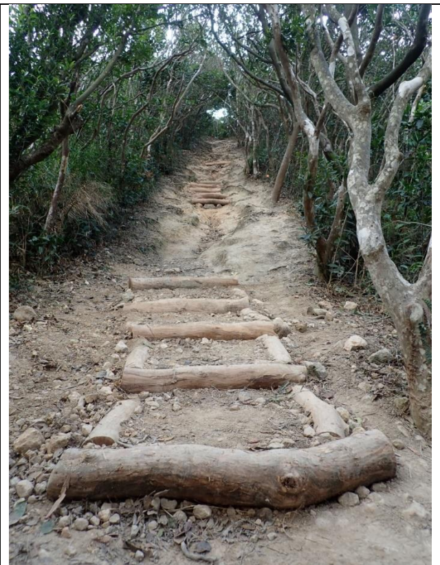
Fig. 2.1.2 Current trails maintenance method
