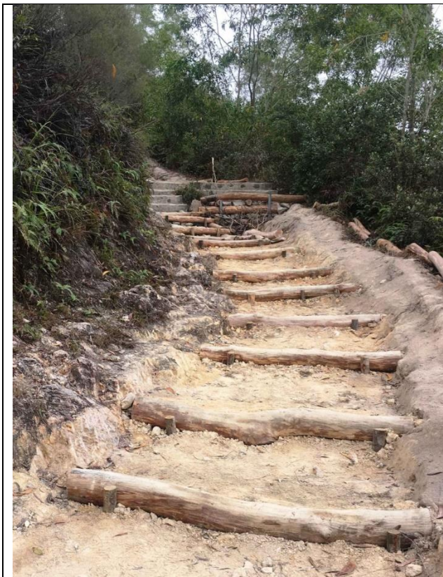
Fig. 2.1.1 Current trails maintenance method
